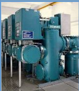
Gas-Insulated Switchgear GIS
