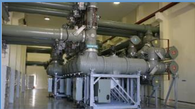
Gas-Insulated Switchgear GIS
