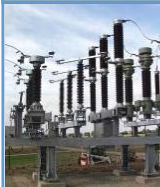
Switchgear Bay SIMOBREAKER
