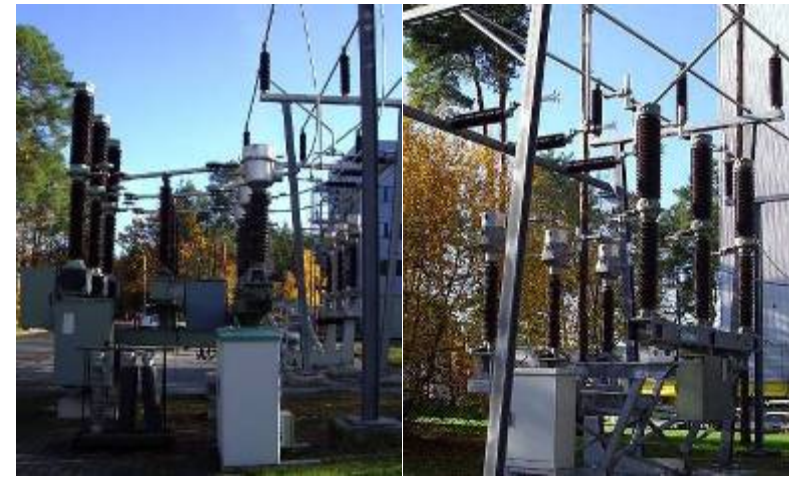
Air-Insulated Switchgear Systems (AIS) All rights reserved Energy / AAN
