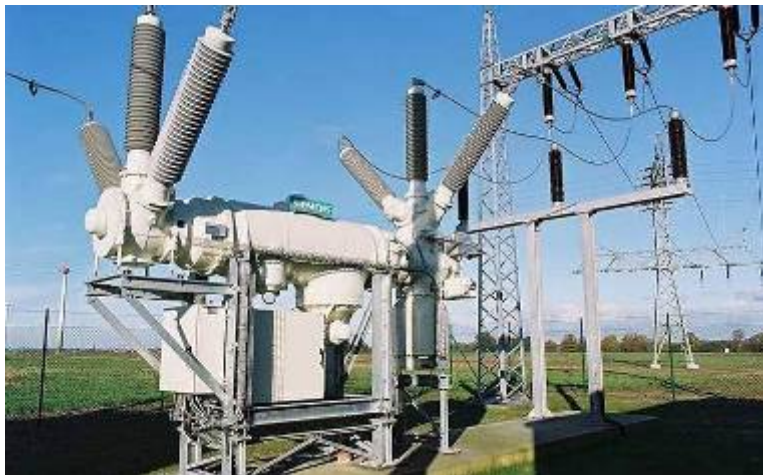
Highly-Integrated Switchgear (HIS)
